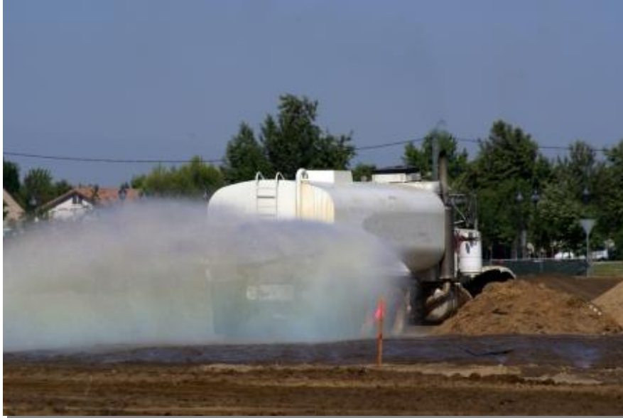
Picture: Water Spraying to Reduce Dust Creation
