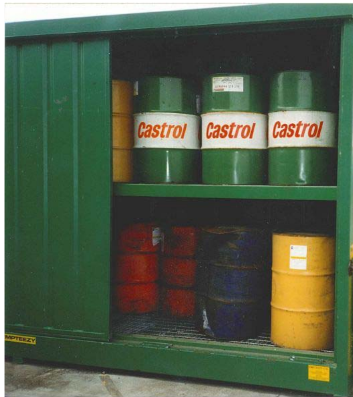
Picture: Effective Containment of Drums
